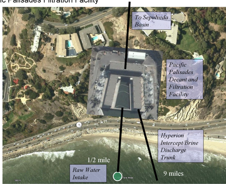
Joseph Jensen Desalination Project Pacific Palisades Filtration Facility
